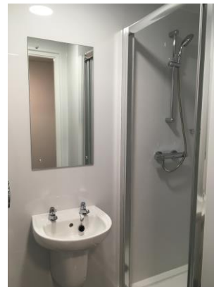
En-suite shower room with hand basin & toilet
